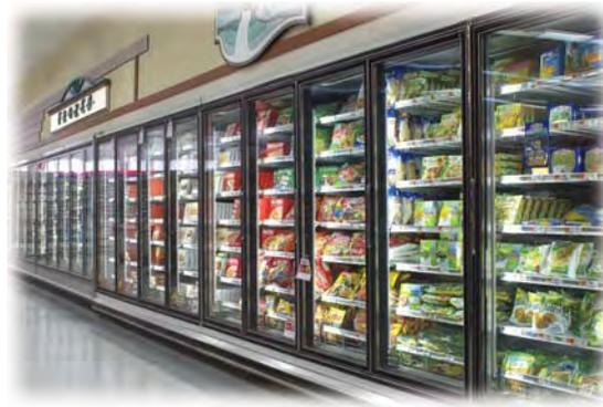
*Energy efficient LED cooler lights and door heaters were installed.*
