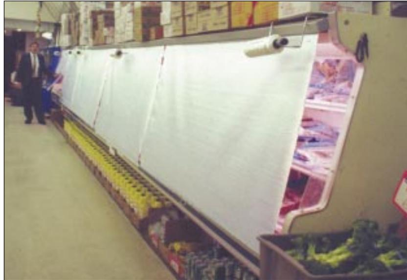
*Aluminum shields reduced infiltration and radiation heat transfer into the display case from the surrounding environment.*
