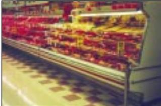
*The tests showed that using the shields during closed hours helped product to stay colder, even though the shields were open during business hours.*
